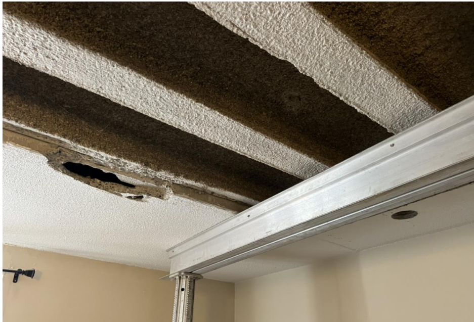
Figure 2: Underside of Precast Panel
