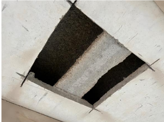
Figure 6: Test opening within Unit 82
