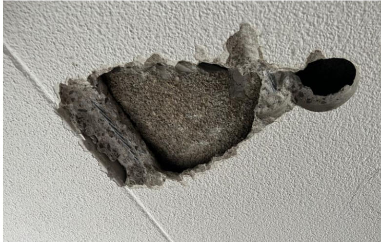
Figure 5: Destructive testing showing no cold joint
