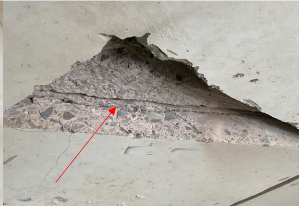
Figure 7: Test opening within Unit 70
