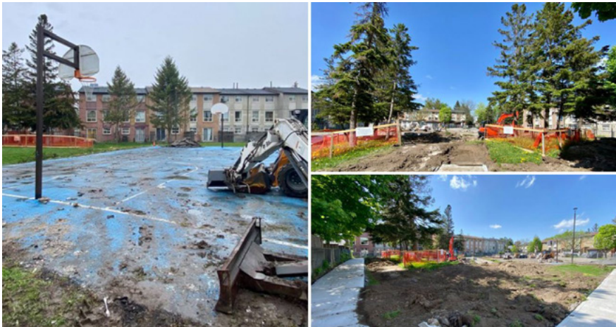
The Empringham basketball court being replaced.
