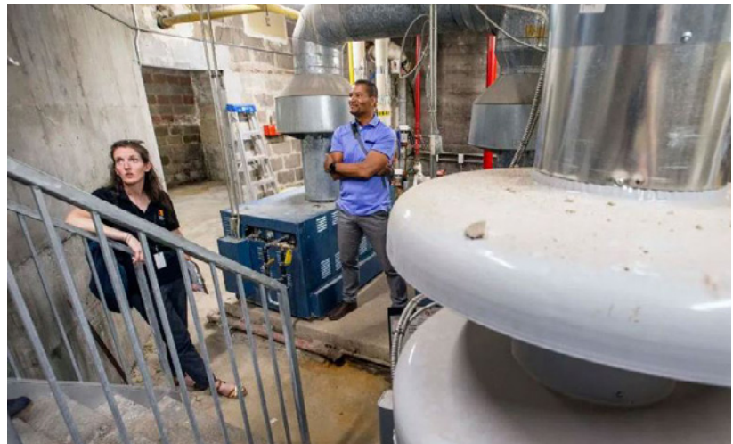
A TCHC building undergoes a green retrofit (photo credit: Toronto Star, June 30, 2022)
