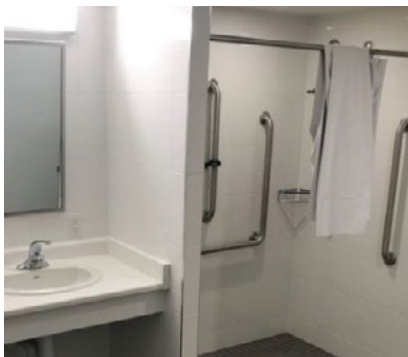
Before and after photos of an accessible washroom modification. Before: step in shower; After: accessible roll-in shower
